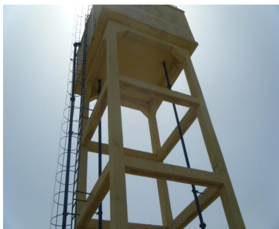
Photo 4: Water tower in the district of Goumori
