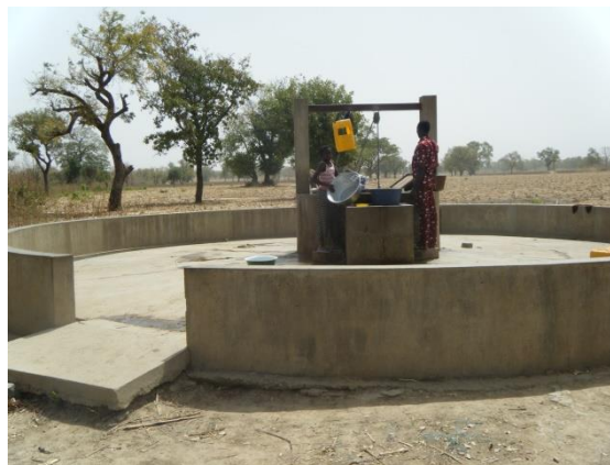
Photo 3: Drilling against well in the district of Gomparou
