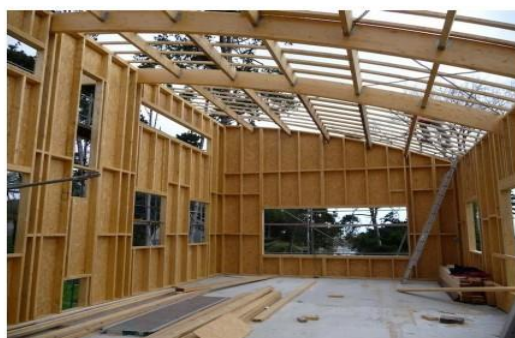
Figure 2. 25: Construction à ossature bois
