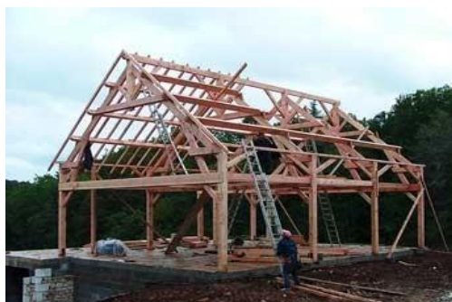
Figure 2. 26: Construction poteaux-poutres
