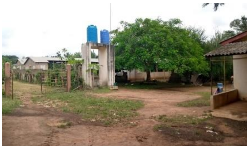
Photo 1: Borehole installed in a farm in Ita-Bolarinwa
