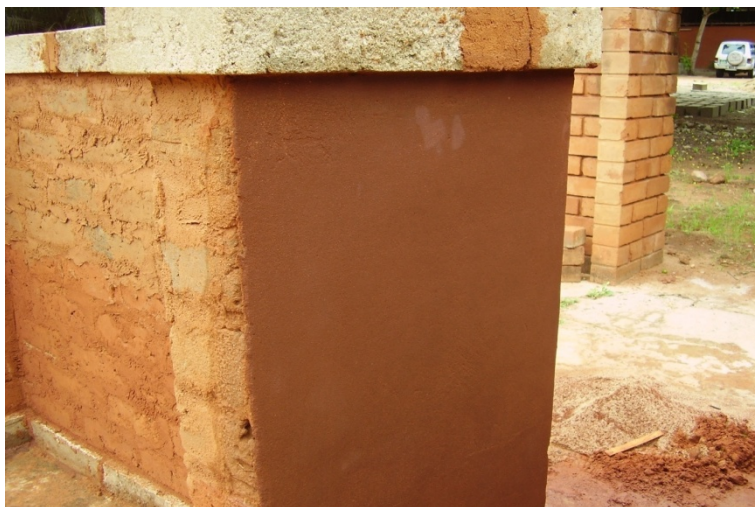
Fig. 4 Clay, sand and locust bean fruit husk's extract.
