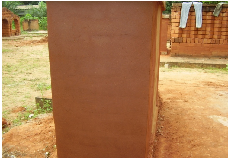
Fig. 2 Micro clay coating, sand and locust bean husk's extract.
