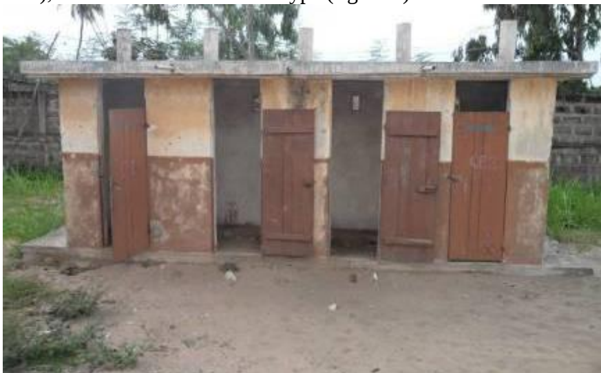
Figure 1. A VIP latrine of 4 cabins equally distributed per gender, in a school of Hilla-Condji, Grand-Popo, July 2013
