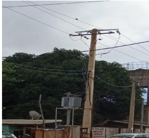
Figure 1: View of the type post on chassis of the Zogbadje district in Benin
