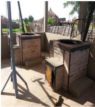
Figure 9. Improved hearth integrated into the GEM system (Dossou, 2015)
